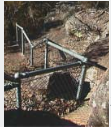
Part of the steep section down to the Galston Gorge bridges
